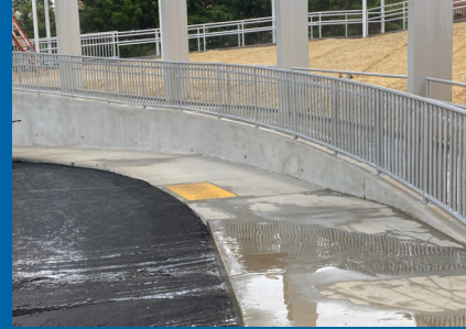
Handrails at Bus Loop ADA Ramp
